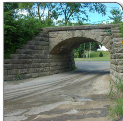
HISTORIC RAILROAD BRIDGE
